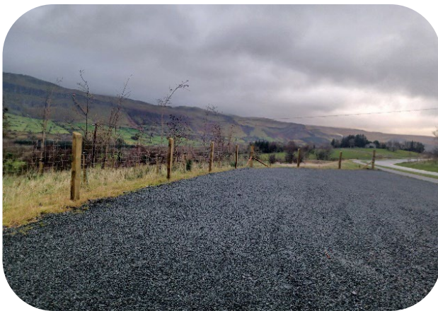
Additional fencing at Collinsford
