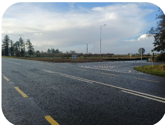
N17 - L 8319 Curry Road Safety Improvement Scheme
