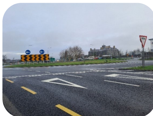
Resurfacing works successfully completed at Summerhill Roundabout to enhance road safety
